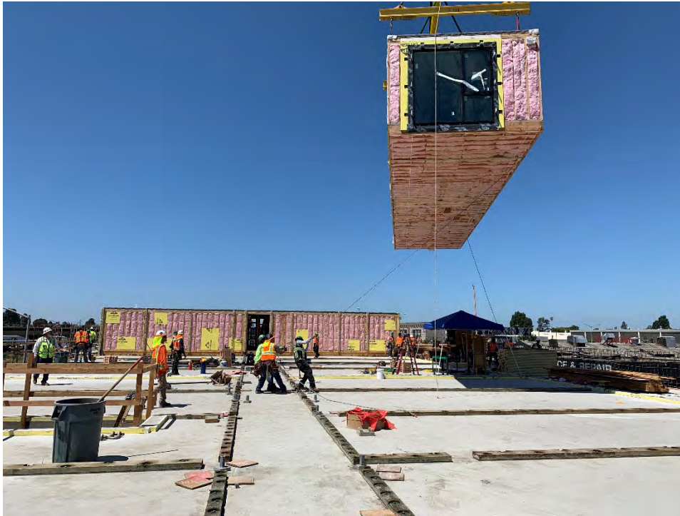
Setting factory-built modules on site-built concrete podium. Image courtesy of Factory_OS.
