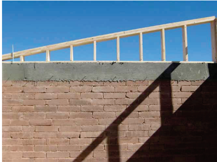
Figure 12. Finished Bond Beam With Shed Roof Framing
