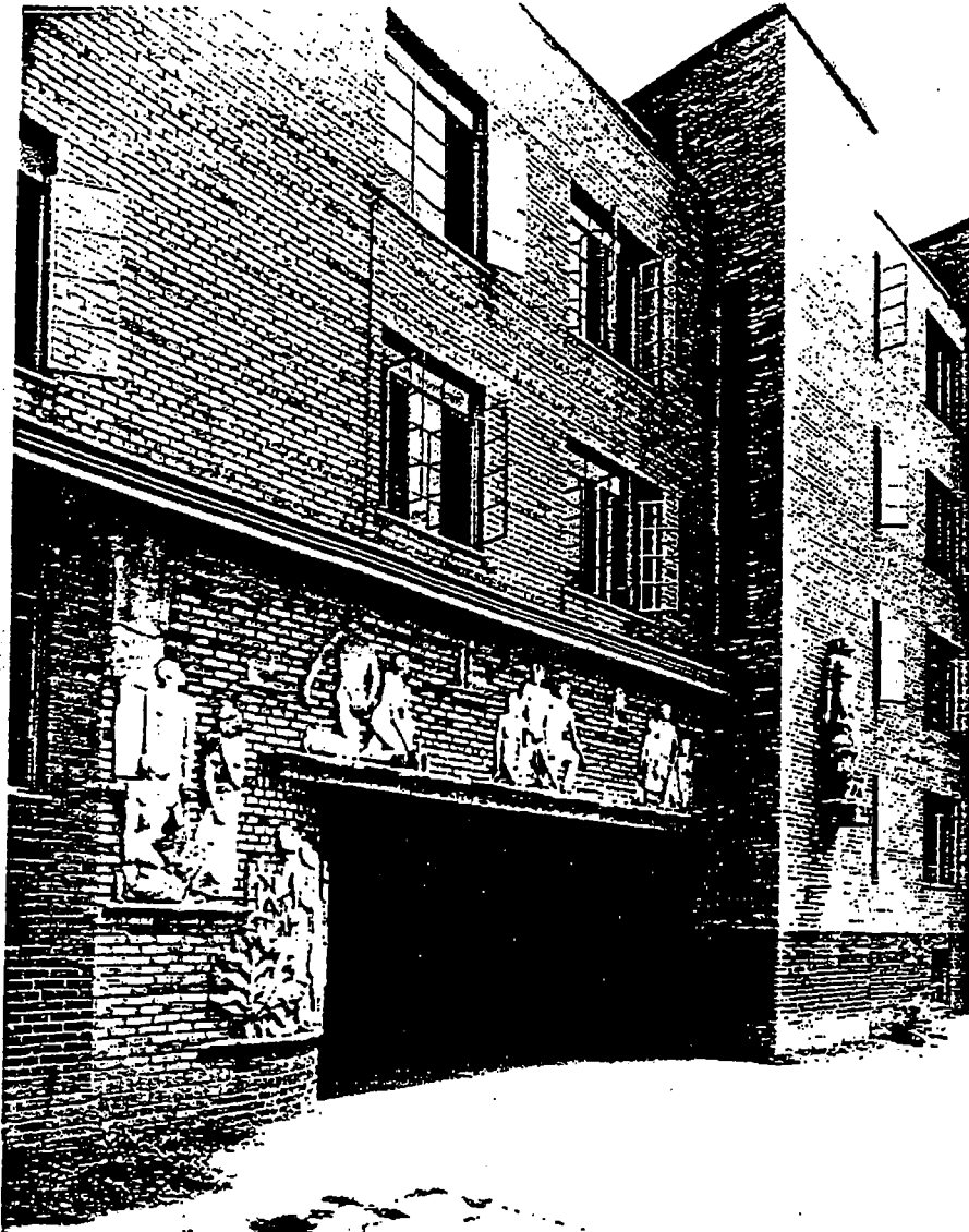
Figure 8 - Detail of building at Langston Terrace in Washington, D.C., a PWA direct-built public housing project completed in 1938, showing typical PWA-era details, including stripped, modern design, brick construction, and casement windows. This complex also featured a significant public art component, a terracotta frieze entitled "The Progress of the Negro Race." (National Register of Historic Places Nomination, 1986)
