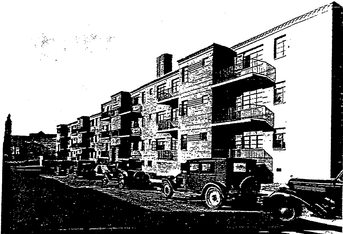
Figure 2 - A representative building at Neighborhood Gardens in St. Louis, Missouri, a PWA limited-dividend public housing project completed in 1935. The 252-unit complex's three-story brick and concrete buildings featured flat roofs and International Style architectural details, common characteristics of the era's early public housing. (National Register of Historic Places Nomination, 1985)
