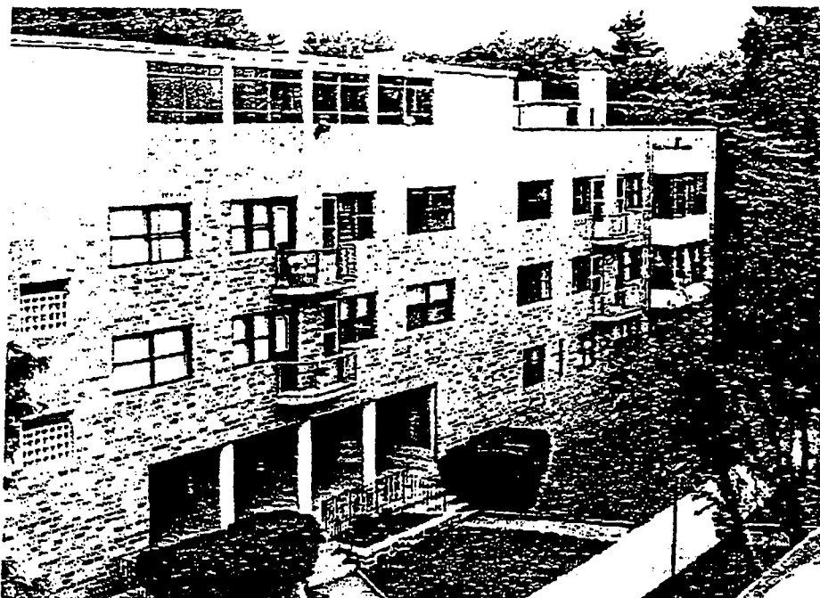
Figure 1 - A representative building at the 284-unit Carl Mackley Houses in Philadelphia, Pennsylvania, the first PWA limited-dividend project completed in 1935. The buildings, covered in burnt yellow and orange industrial tiles, were particularly modern in appearance. (National Register of Historic Places Nomination, 1998)
